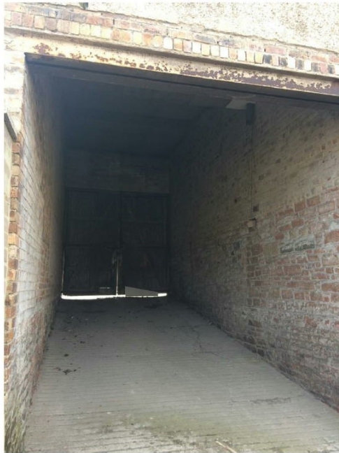
Existing Pend/Vehicular Access (viewed from courtyard area)
